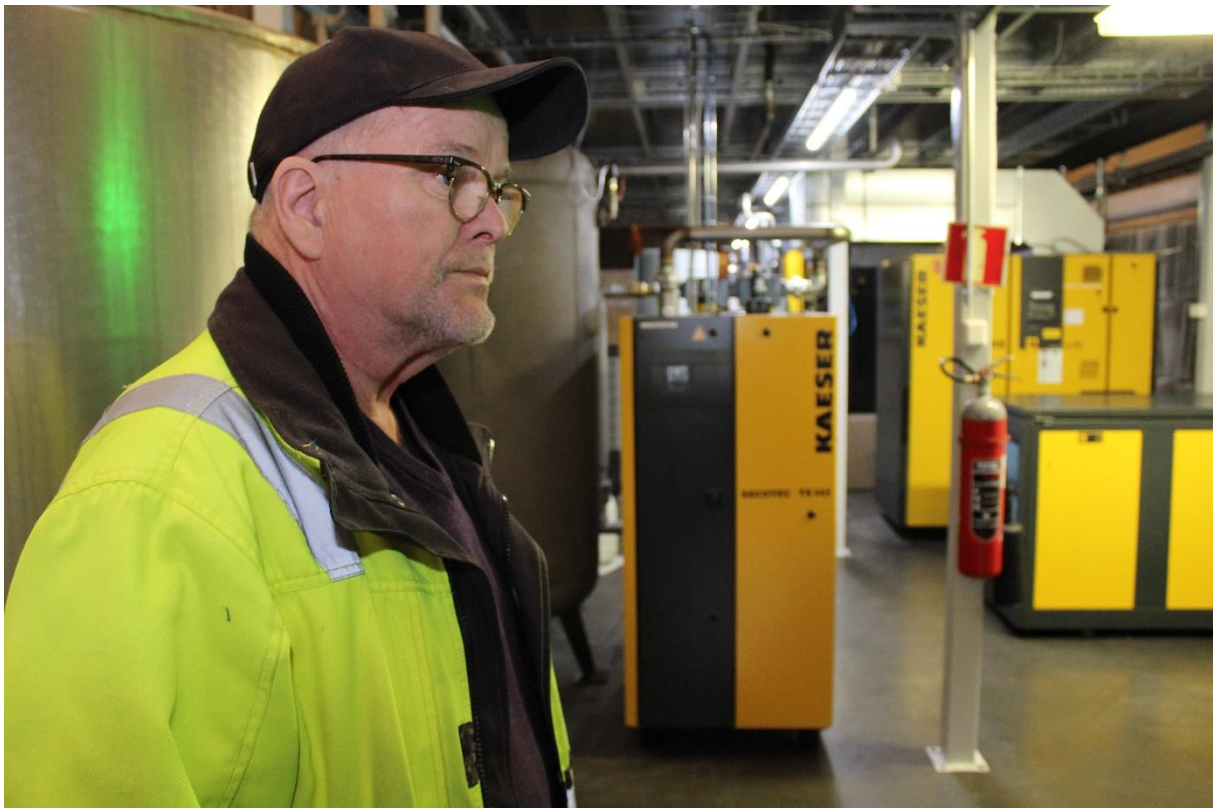
The production chief Jari Myllykangas is satisfied with the system at Finn Spring that stored waste heat from the factory compressors to the ground to be used later.
