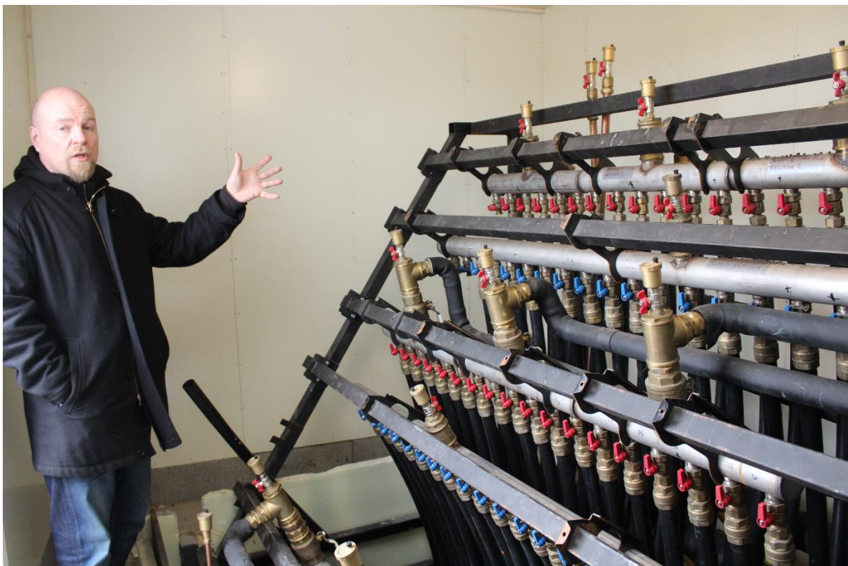
Timo Sivula shows the controller house, where the tubes to the BTES are collected. The tubes transport waste heat and the heat from the solar thermal collectors to the ground.
