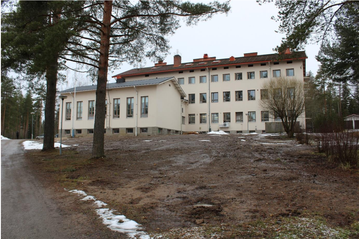
The boreholes for geothermal heating and seasonal storage in front of the school.
