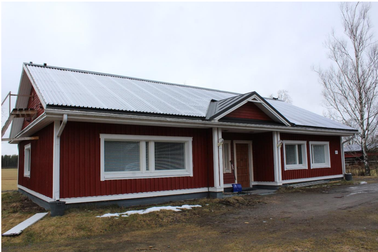
Solar thermal collectors on a roof of a detached house in Sokoja.
